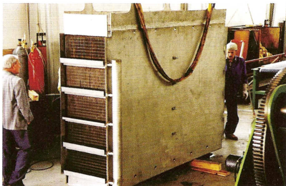
Fig. 1: Evaporator in Waghäusel under construction
